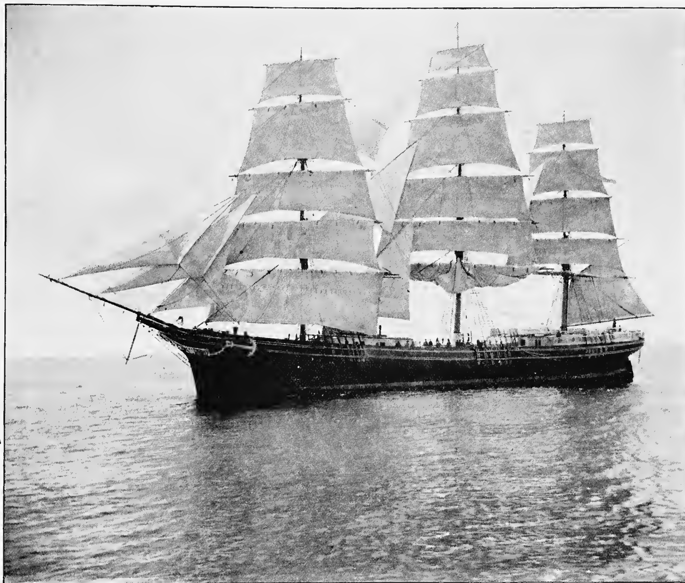
THE GRANITE STATE.—A Typical American Wooden Sailing Ship.
